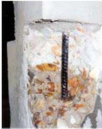
Damp the surface
