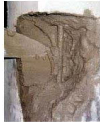
Apply the mortar
