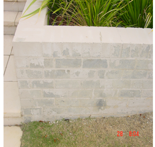
To repair flaking, peeling previously painted surfaces.
