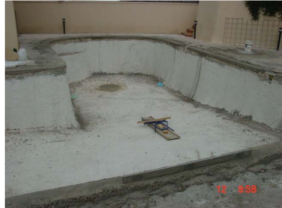
The bare concrete shell.
